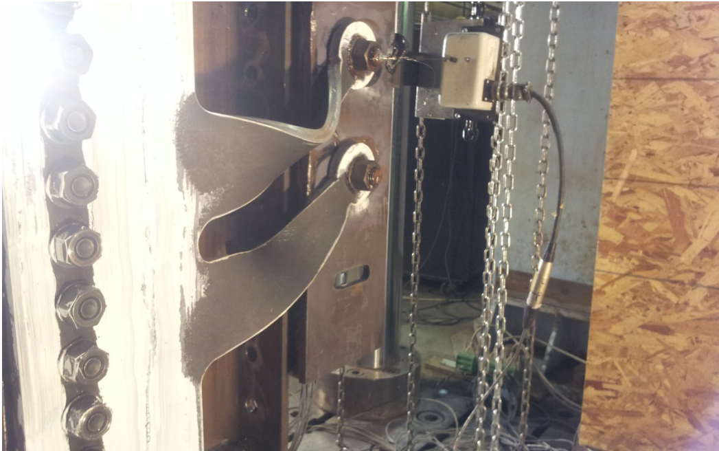
Figure 5-12: Test Specimen # 1 – Buckling of Steel Fuse Plate – Cycles 11 and 12
