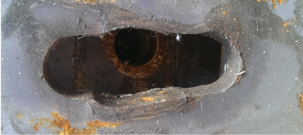
Figure 5-16: Deterioration of Slots within Fuse Attachment Plate
