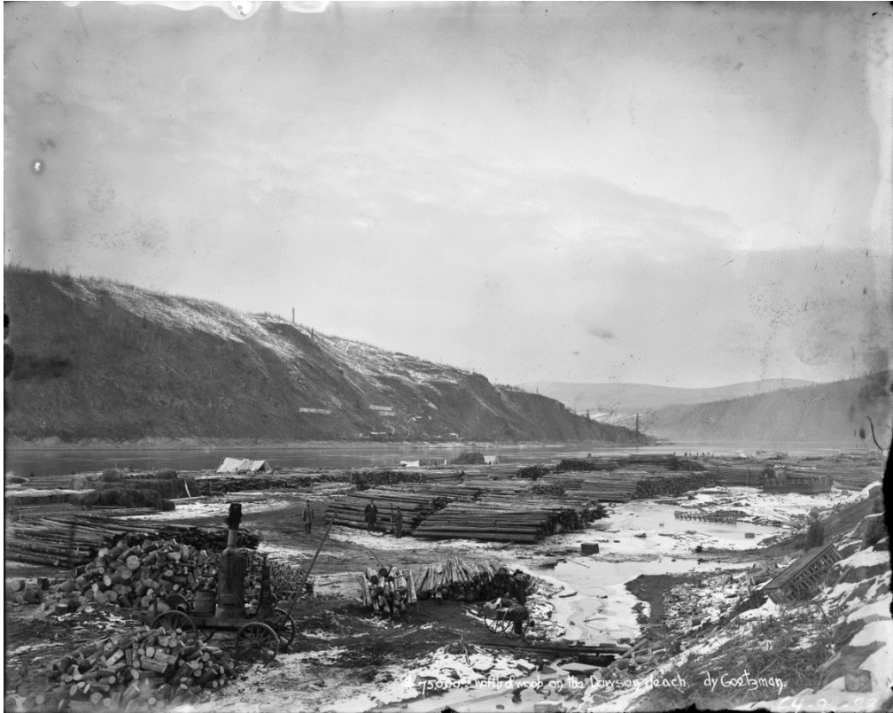
Image 4.1 A pile of wood near Dawson City reportedly worth $750, 000 at the time, thought to be early 20 th century. University of Alaska Fairbanks Archives. Selid-Bassoc Photography Collection 1964-92-382
