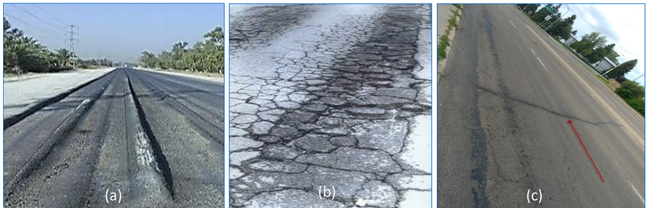
Figure 2-1: Common distresses (a) Rutting- permanent deformation (b) Fatigue cracking (c) Low temperature cracking
