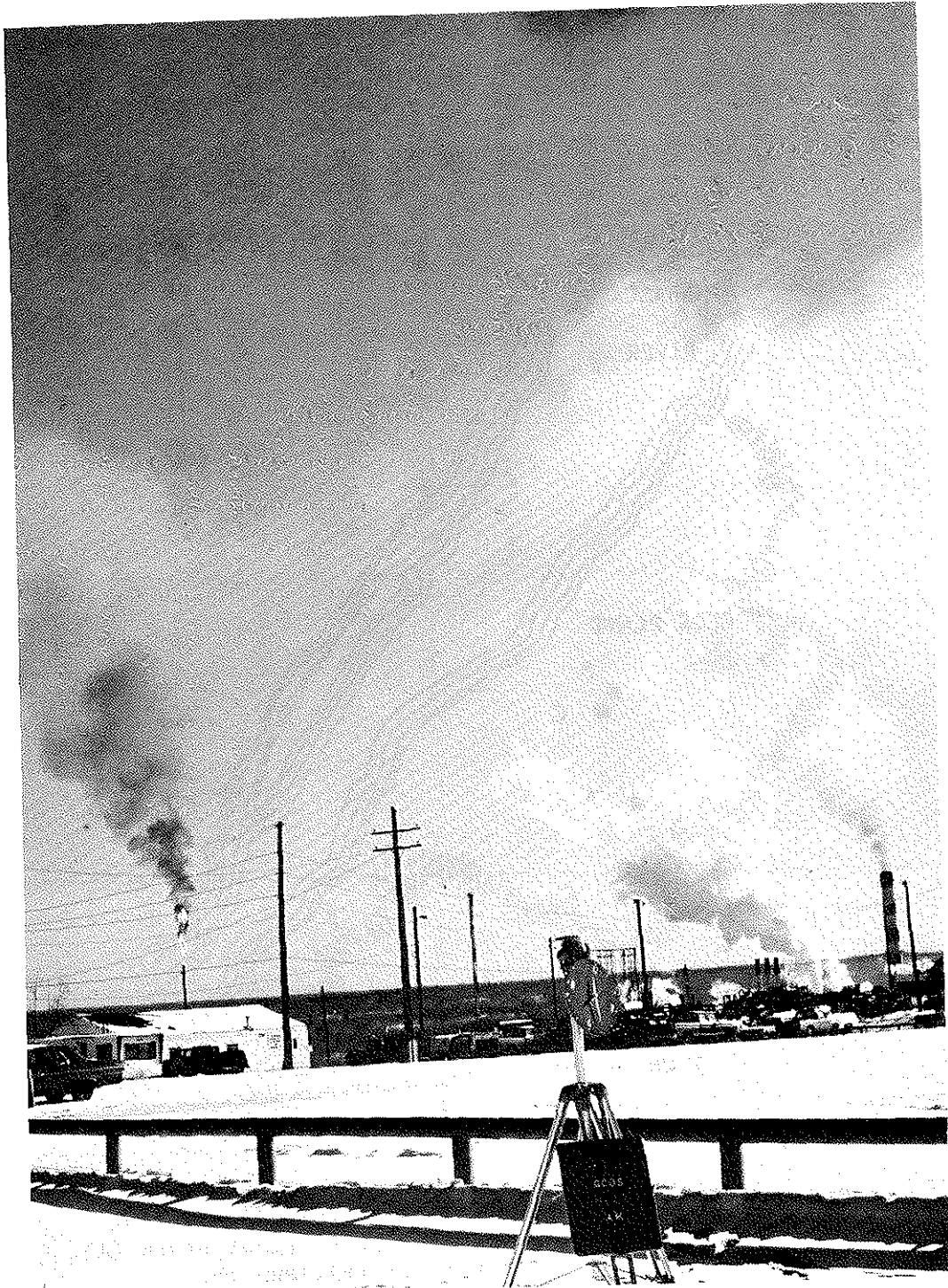
Figure 5.2. The GCOS plant in operation.
