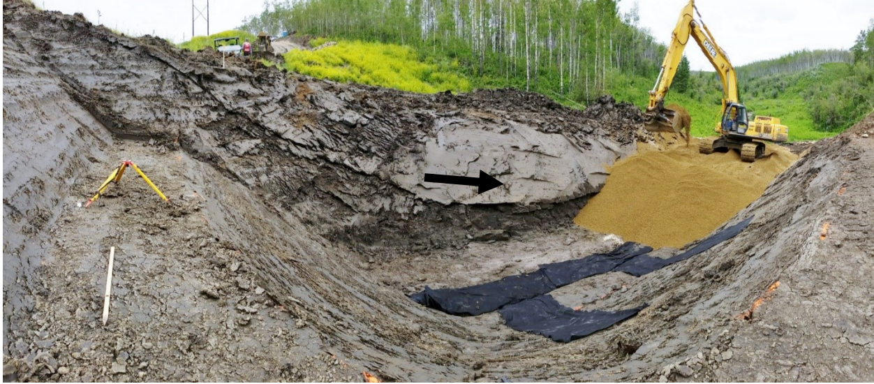
Figure 3.15: A slip surface can be seen during panelled construction of a granular shear key (McLachlan, 2016). The direction of sliding is indicated by a black arrow. Photo by Duncan McLachlan. Used with permission.
