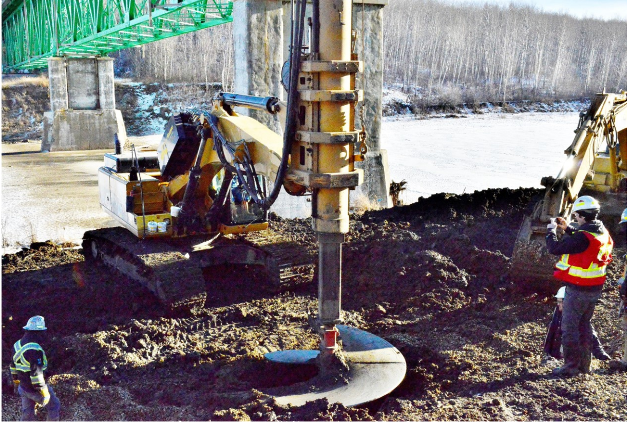
Figure 2.13: A large-diameter auger being used in the installation of a rockfill column along a riverbank underneath a bridge. Photo by Hugh Gillen.
