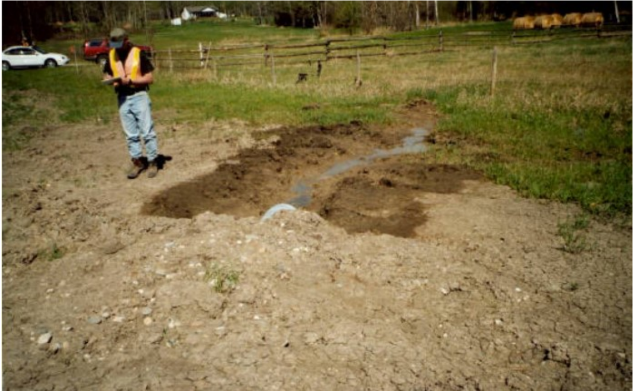
Figure A-26: Continuous flow coming from the outfall pipe draining the granular toe key (Tetra Tech EBA, 2002). Reproduced with permission from Alberta Transportation.
