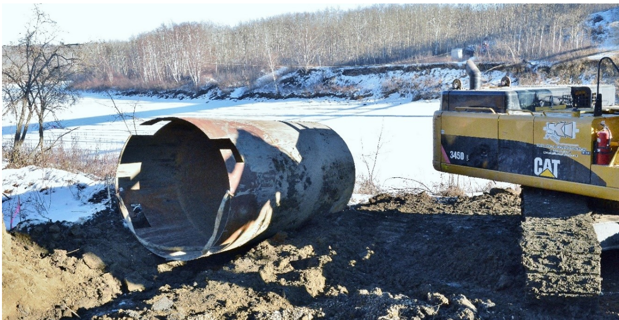
Figure 5.1: A steel sleeve used to help maintain hole stability during the construction of rockfill columns. Photo by Hugh Gillen.
