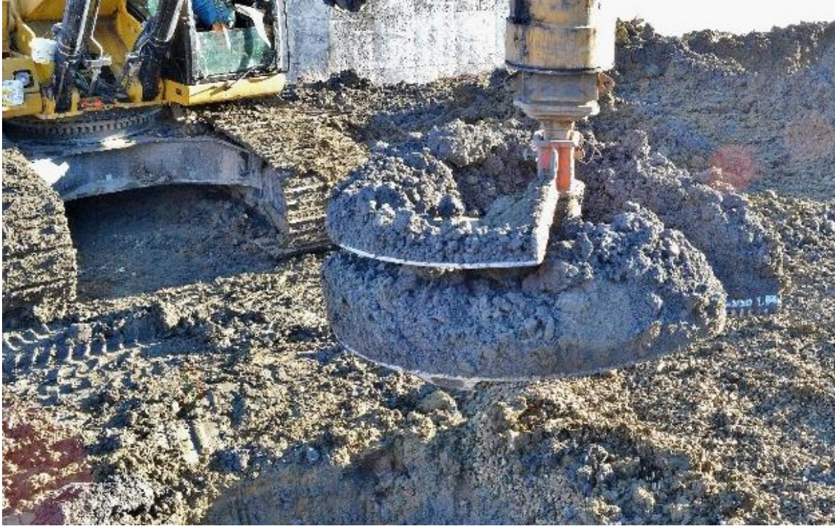
Figure 3.17: Pictured is a 2.13 m diameter auger in the process of lifting soil from a hole that is being excavated for a rockfill column. Photo by Hugh Gillen.
