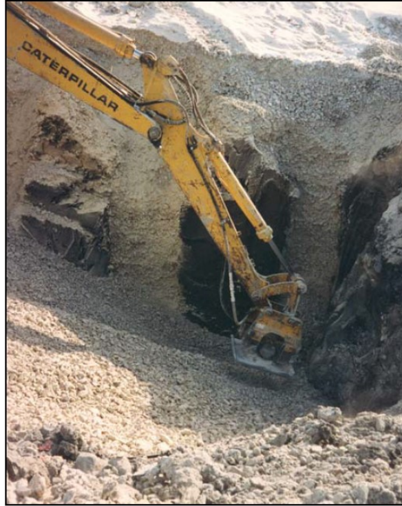
Figure 3.16: Shear key backfill being compacted with a vibratory plate. Reproduced from Yarechewski and Tallin (2003), with permission.
