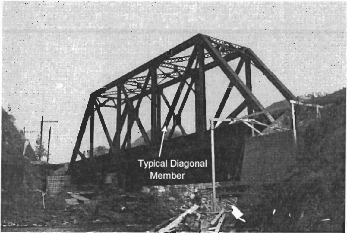
Figure 3.1 Bridge in Service
