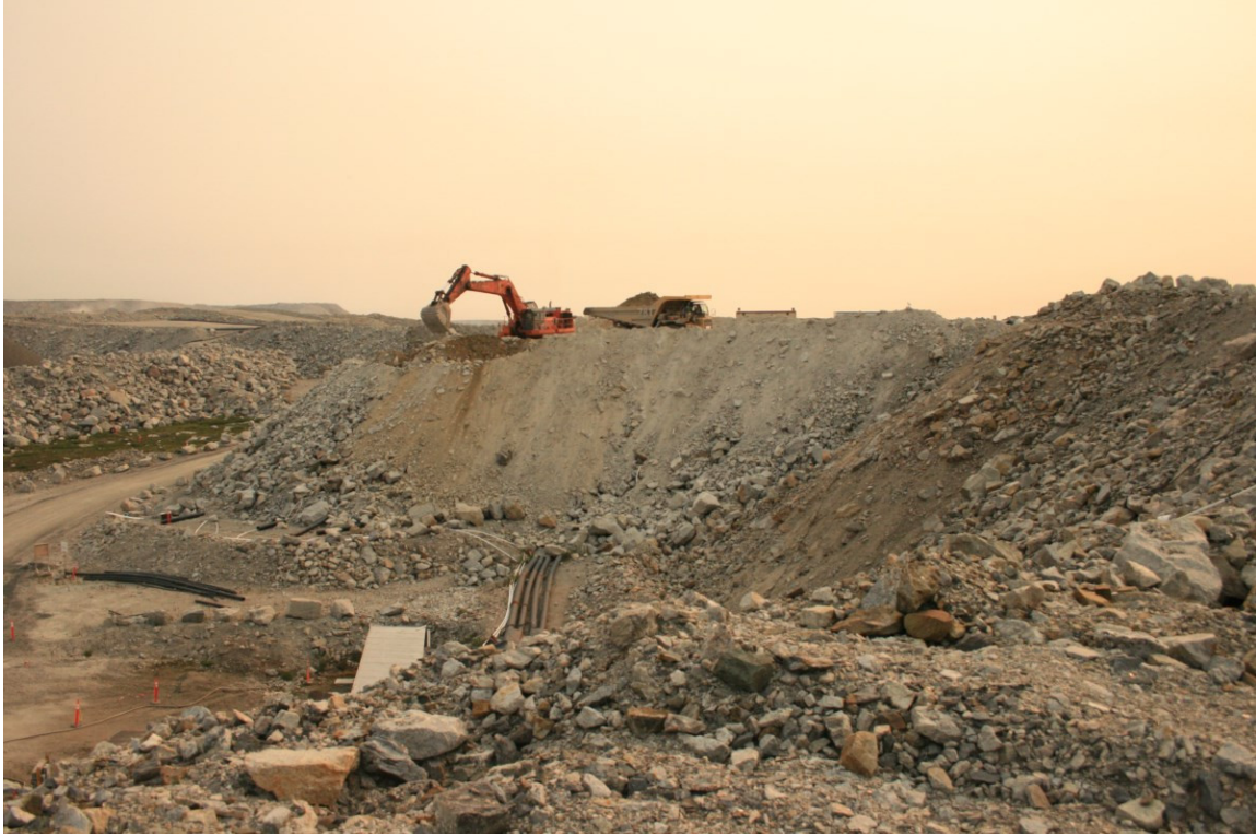
Figure 6 - Type I test Pile During Deconstruction (July 3, 2014)
