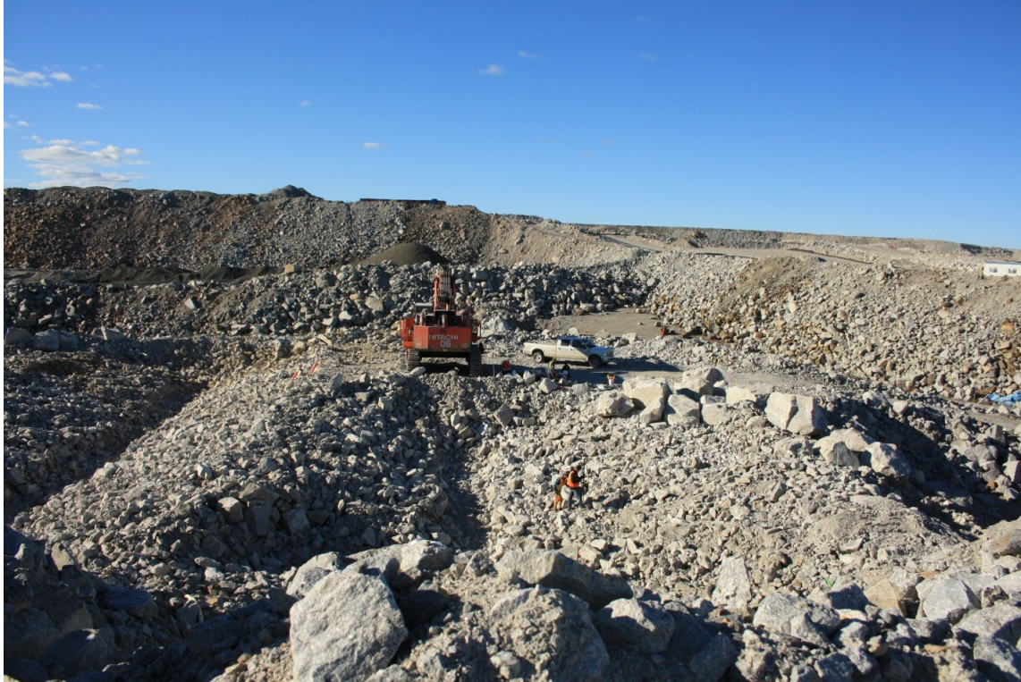
Figure 10 - Deconstruction of the Type I Test Pile
