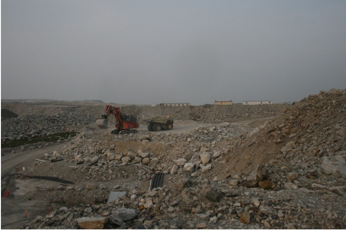
Figure 8 - Type I test Pile During Deconstruction (July 28, 2014)
