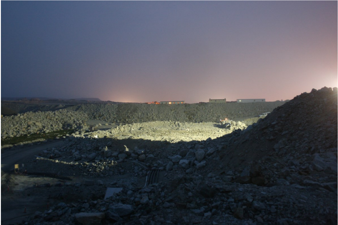
Figure 9 - Type I test Pile During Deconstruction (August 2, 2014)
