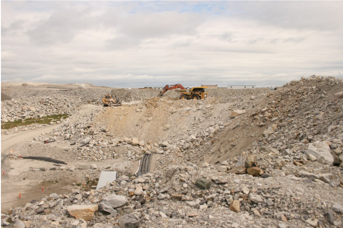
Figure 7 - Type I test Pile During Deconstruction (July 7, 2014)
