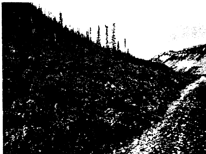
Fig. A .7 Mile 120.7 Dempster Highway (Ten ft. cut with 2:1 backslopes made into ice rich organic silt.
