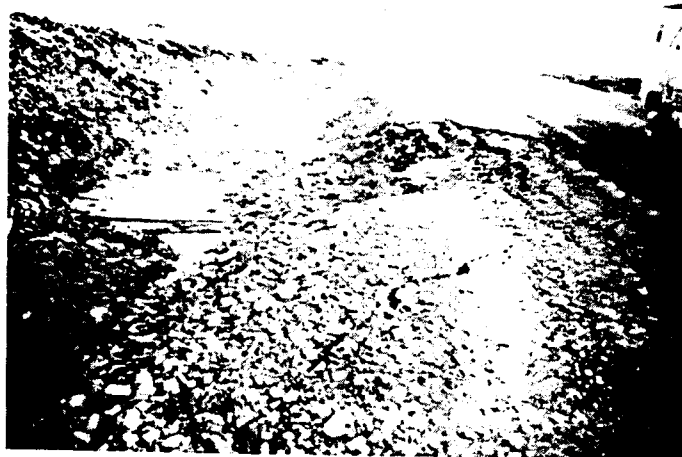
Fig. A.10 Mile 175 Dempster Highway (Backslope and shoulder failure due to melting of a large ice lense).
