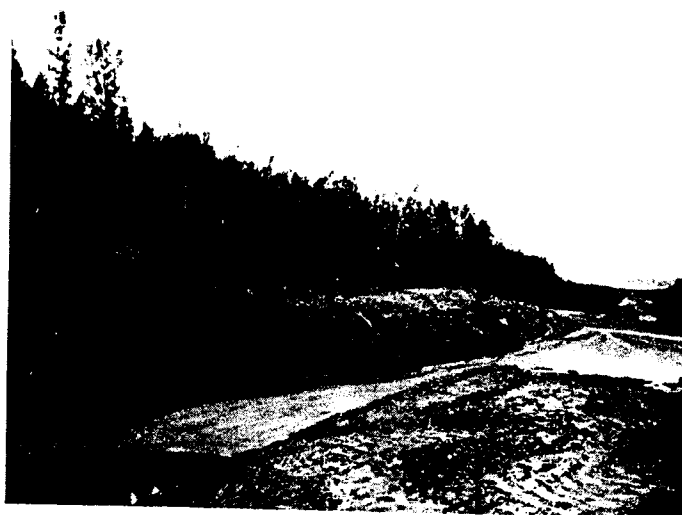
Fig. A.1 Mile 222 Alaska Highway (Backslope instability during construction, July 1973).
