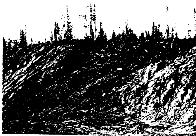
Fig. A.13 Mile 343 Dempster Highway - Stabilized backslope. (Hand placed vegetation to control rate of thaw).
