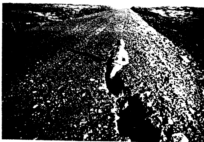
Fig. A.11 Mile 175 Dempster Highway (Severe cracking of shoulder due to differential thermal subsidence caused by construction).
