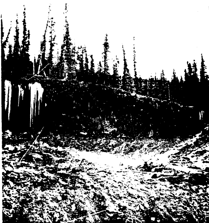
Fig. A .8 Mile 153 Dempster Highway (Melting of large ice wedges caused slope degradation).
