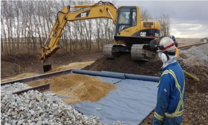
Figure 3.11. Sub-ballast placement over geotextile on April 23, 2019 (Abdulrazagh 2019 – with permission).
