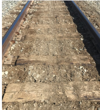
Figure 1.3. Track conditions at the research site before renovation (Abdulrazagh 2019 – with permission).
