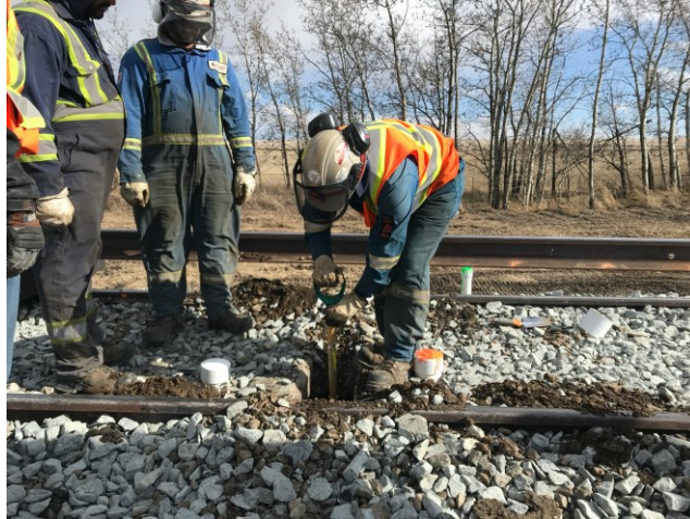
Figure 3.14. Trench boring for access pipe on April 24, 2019 (Abdulrazagh 2019 – with permission).
