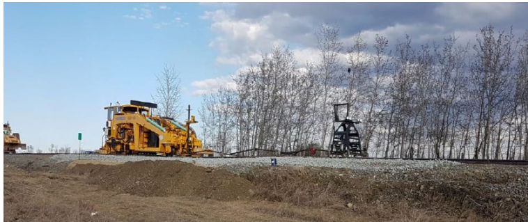
Figure 3.13. Harsco equipment tamping and lining the track on April 24, 2019 (Clifton Associates, 2019).
