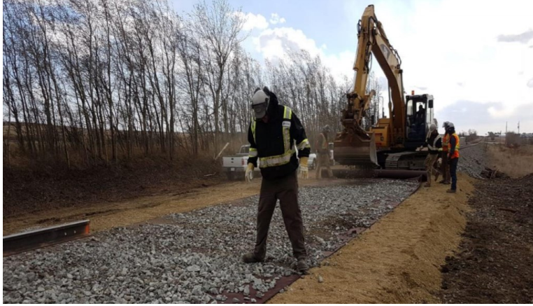
Figure 3.12. Mirafi® RS580i over compacted sub-ballast layer on April 23, 2019 (Abdulrazagh 2019 – with permission).
