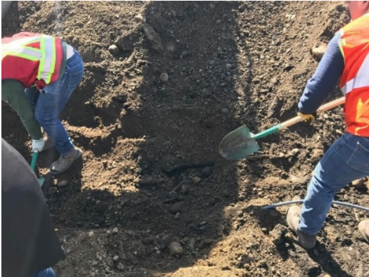
Figure 3.10. Subgrade sensor buried with an electric shield on April 23, 2019 (Abdulrazagh 2019 – with permission).
