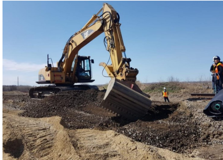
Figure 3.9. Track Section Excavation on April 23, 2019 (Abdulrazagh 2019 – with permission).
