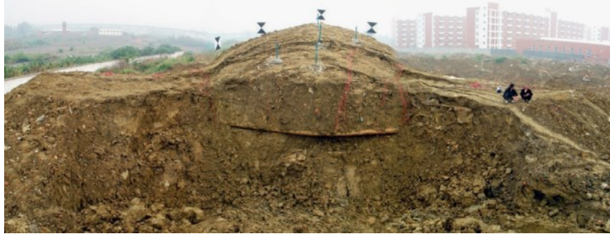
Figure 1-12: Full view of the landslide and pipeline model in Feng et al. [64]
