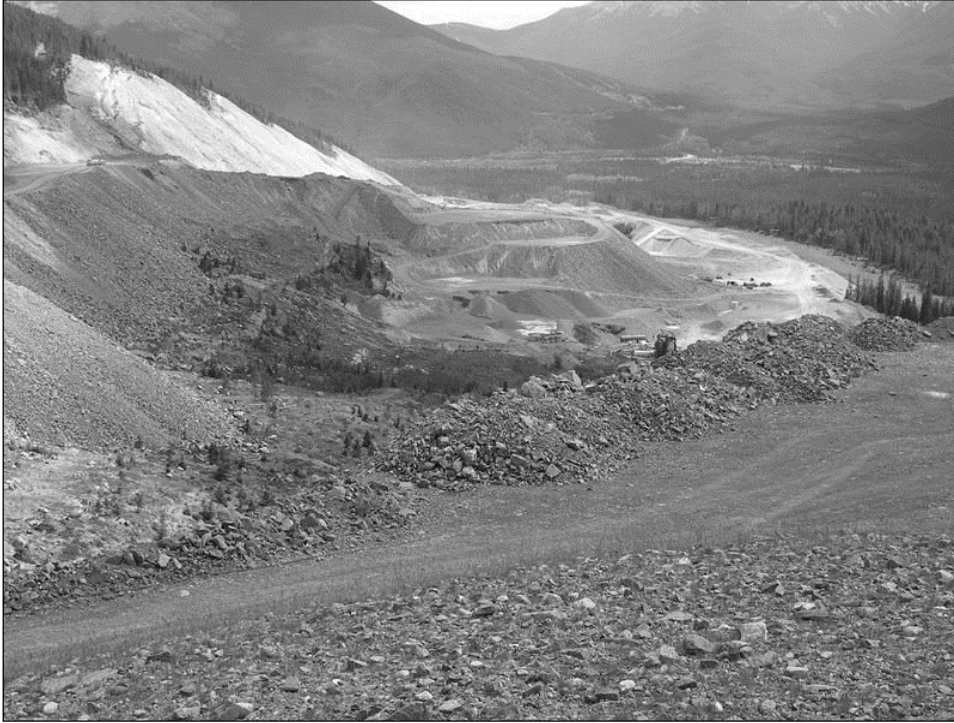
Figure 1-1. View of the Exshaw quarry, Alberta, Canada.
