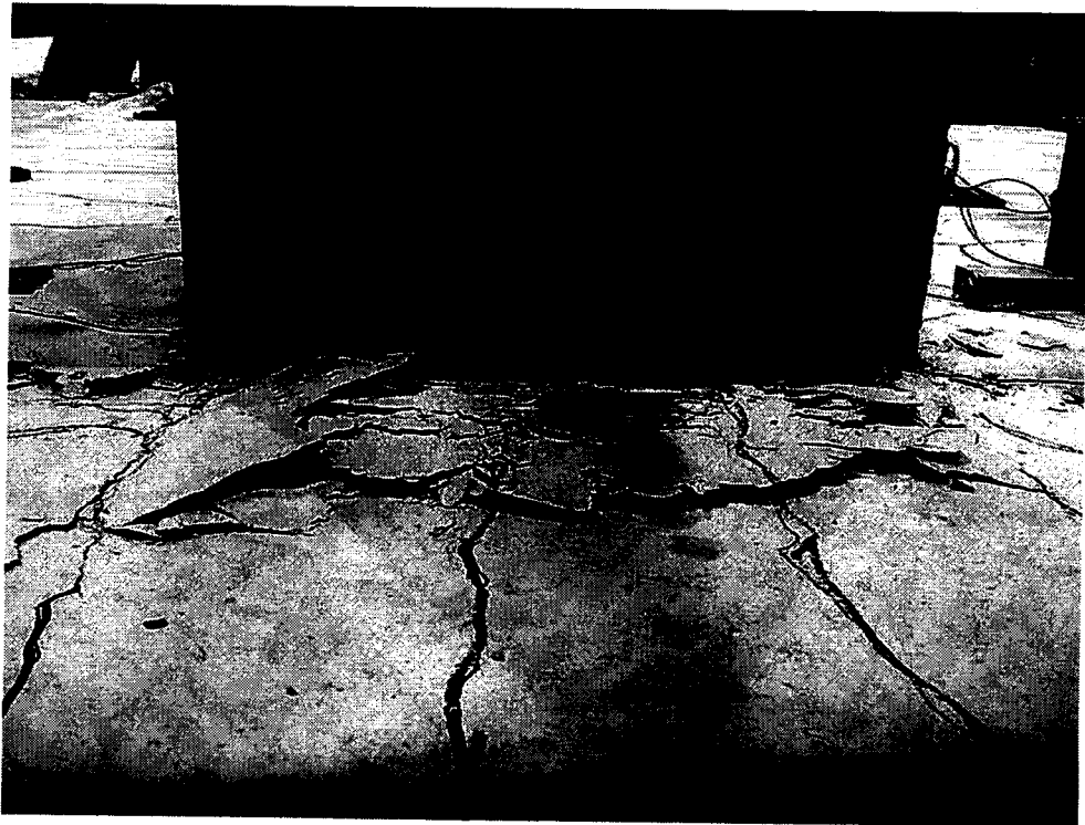
Figure 4.39 (b) Failure Surface of Sp-A
