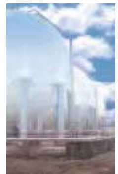
Our Augusta nitrogen plant is ISO 9001 certified.
