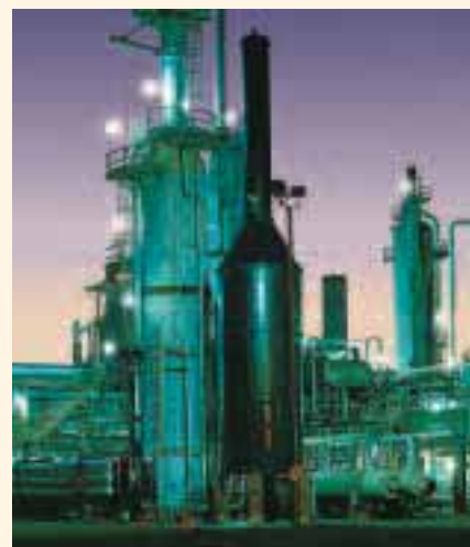
All four ammonia plants at our Trinidad facility are undergoing debottlenecking expansions.
