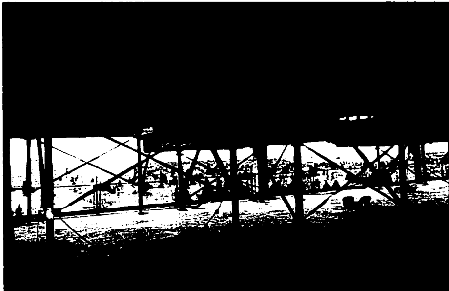
Figure 5-3 Slab Fly Forms Used For ECERF Building Floor Construction
