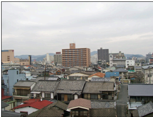
Figure 11. Older residences in Kurashiki, with more recent buildings in the background.
