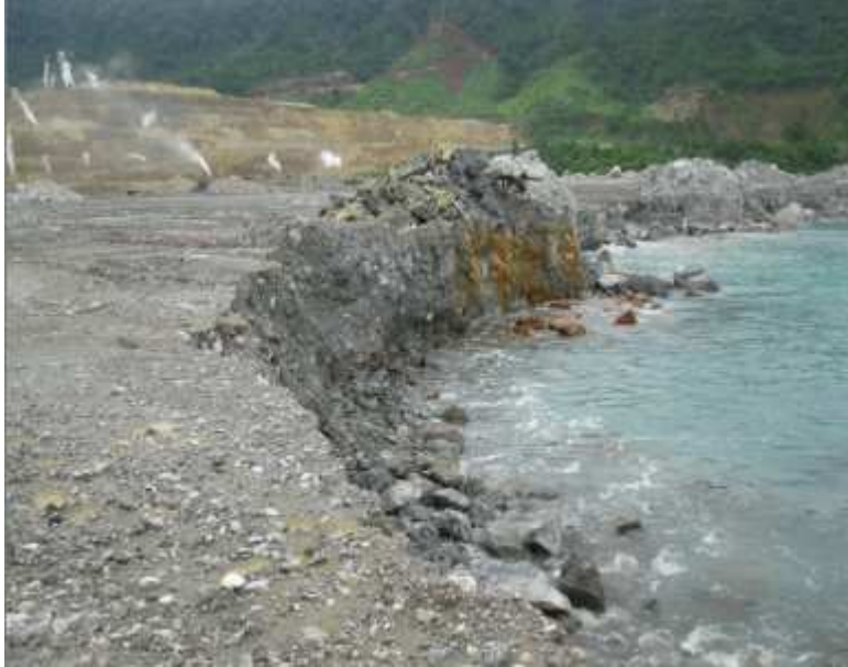
Figure 31: Harbour Base 501 waste dump failure (Lihir Gold Ltd)
