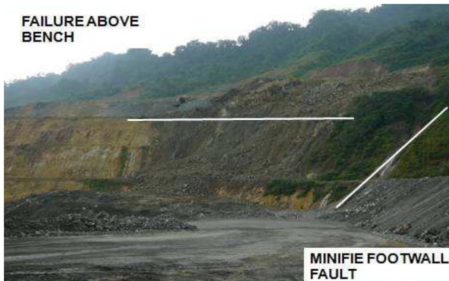
Figure 18: Southern failure bounding structure
