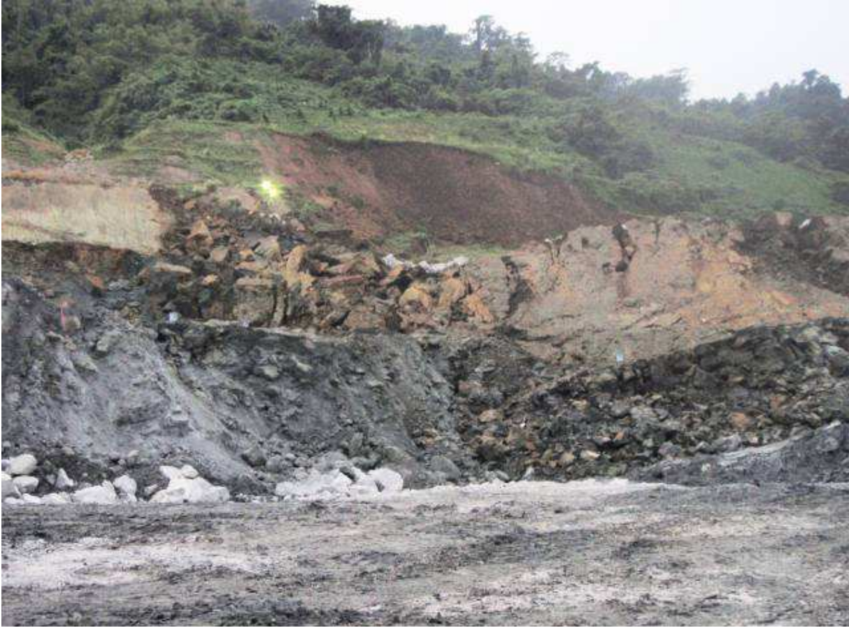
Figure 16: Northern failure margin
