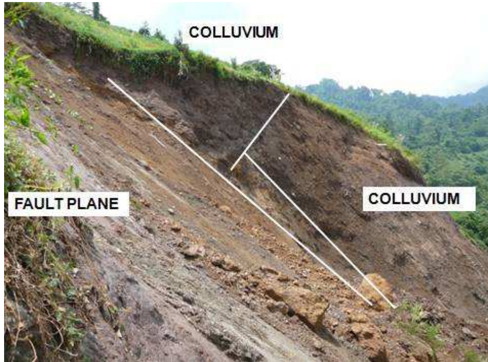
Figure 17: Failure back scarp
