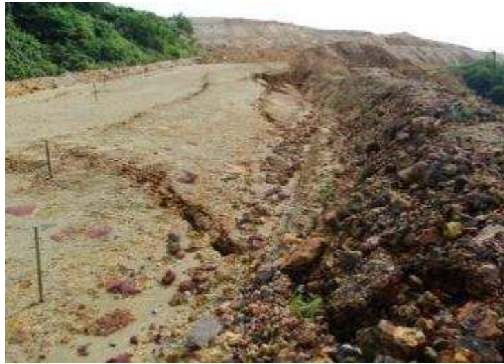
Figure 30: Cracking of Kapit 6 ramp haul road (Lihir Gold Ltd)
