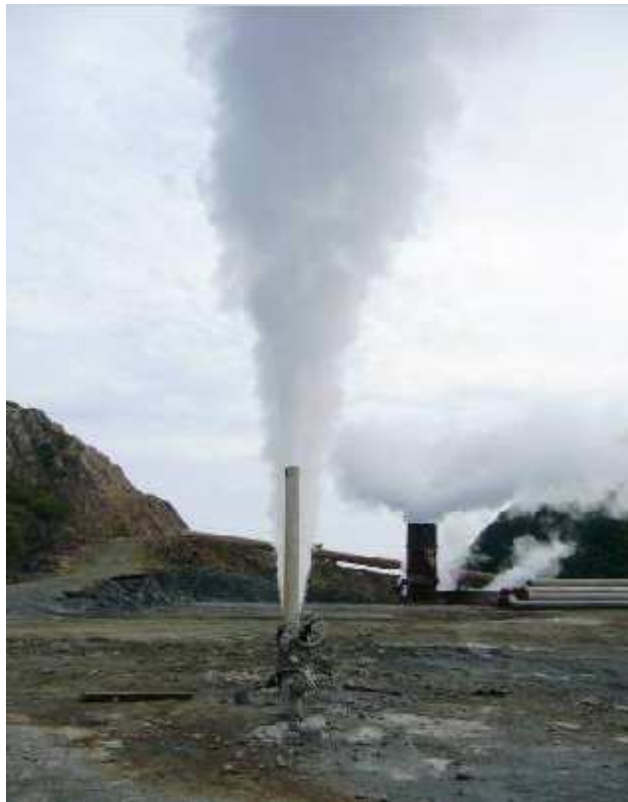
Figure 41: Steam relief wells on Kapit stockpile
