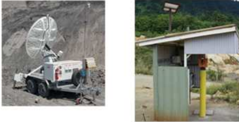
Figure 27: Slope stability radar and robotic theodolite
