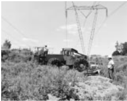
Application of selective herbicides in a power line right-of-way
