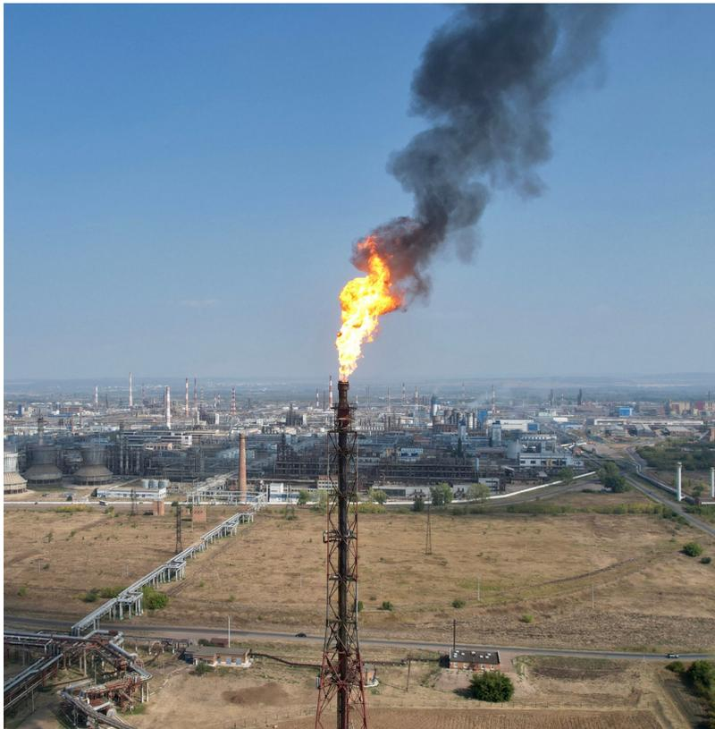
Figure 1.1: Flare stack with smoking flame in a mild crosswind, source of the image (GGFRP, 2022).
