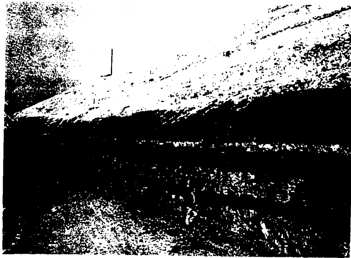
Plate 2.1 View of the east abutment core trench at Boundary Dam Saskatchewan. Note the three separate coal layers and the upwarping of the beds towards the valley. ( Courtesy of P.F.R.A. )
