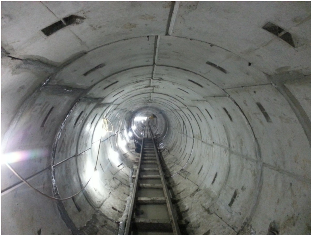
Figure 6-1 A Storm Tunnel under Construction Using Segmental Concrete Liner in Edmonton
