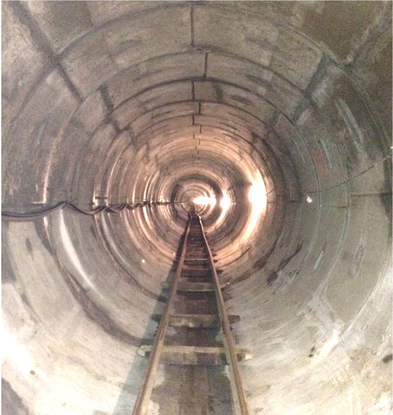
Figure 6-10 Tunnel after “Reinforcement” Removed
