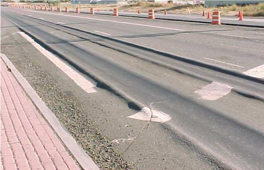
Figure 2.6 Sever rutting in the pavement (Pavementinteractive.org, October 2012).
