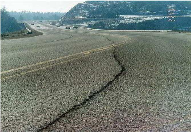
Figure 2.4 Wheelpath (load induced) longitudinal cracking (Pavementinteractive.org, October 2012)
