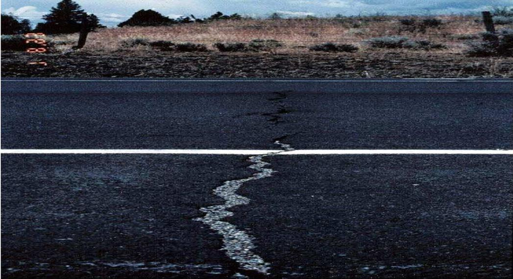
Figure 2.5 Picture of a high-severity transverse crack (Pavementinteractive.org, October 2012)
