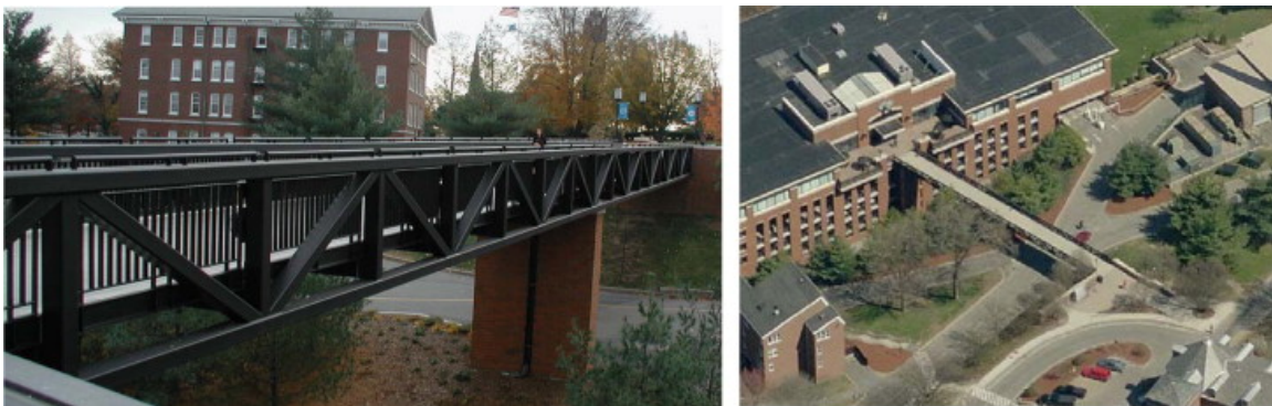
Figure 4.1. Dowling Hall Footbridge (from Moser and Moaveni 2011 with permission)
