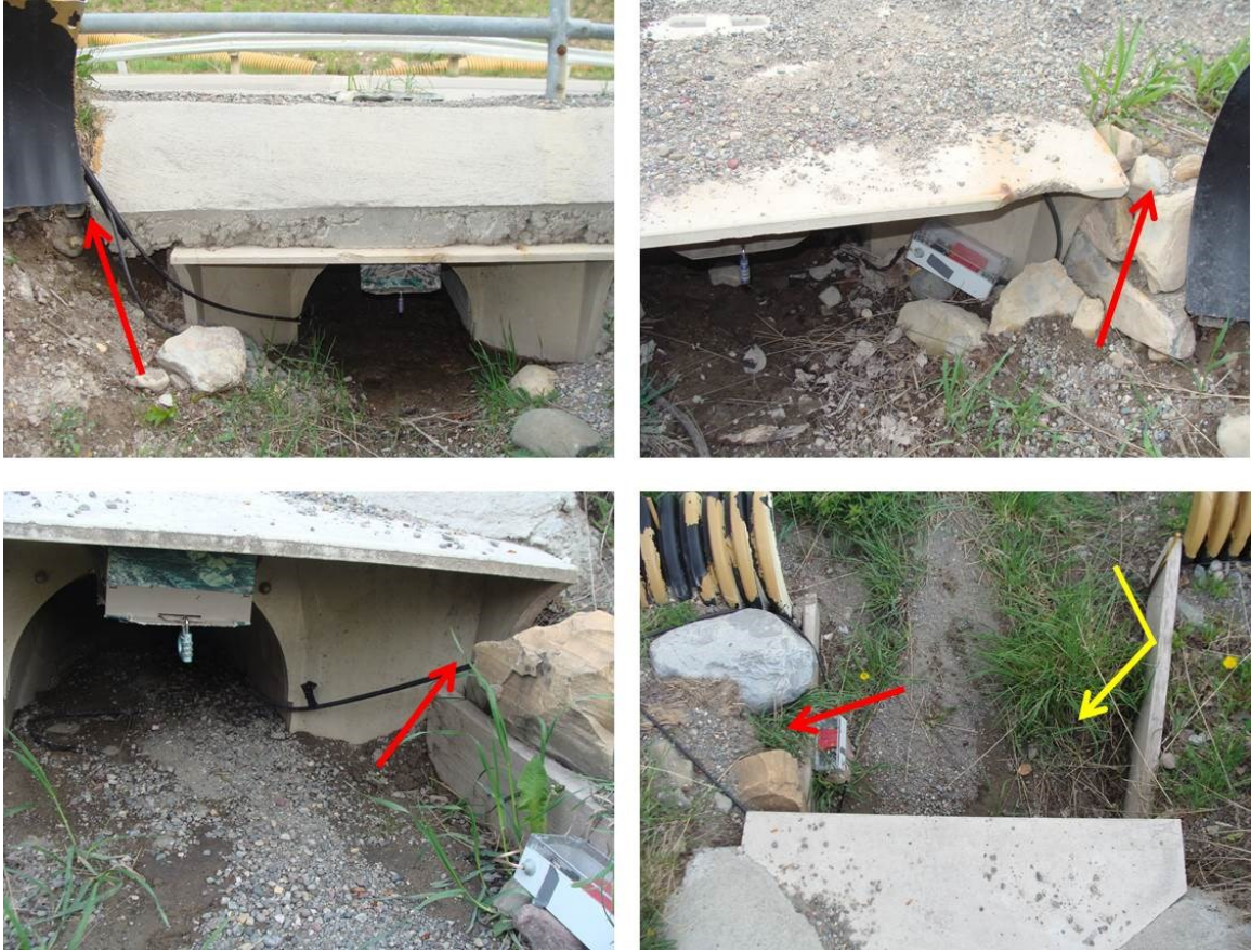
Figure 2.11 Examples of locations where salamanders could bypass the fence-tunnel system at junctions of fences and tunnels. Red arrows show possible “escape routes” and yellow shows a well-designed junction.
