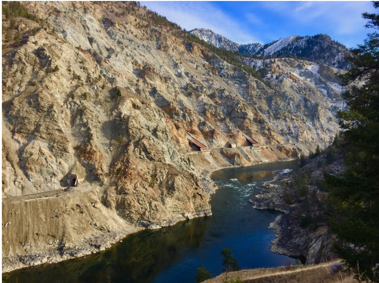
Figure 3: Rail traffic in the Fraser Canyon, B.C. Note the presence of structures to deflect rockfalls over the track and the complex geometry of the slopes generating and deflecting rockfalls. (Photo courtesy D. Bonneau, 2019)
