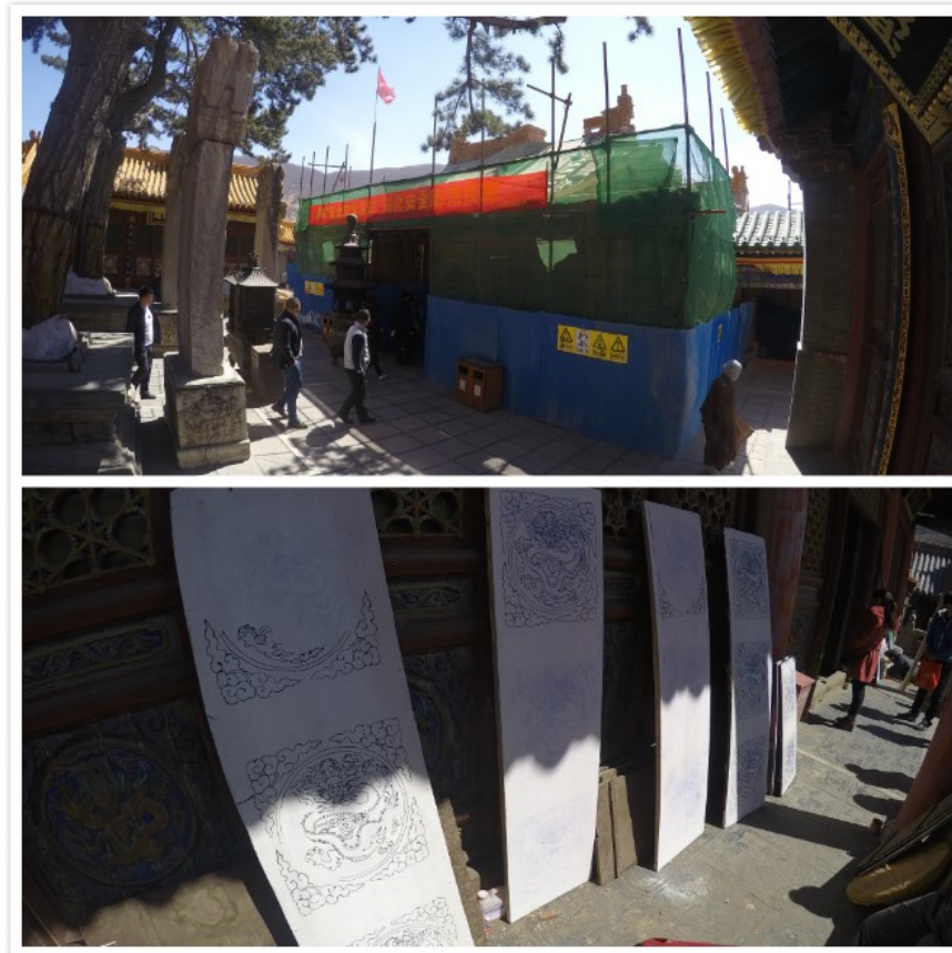
Figure 19: Repairing work at Pusa Ding
