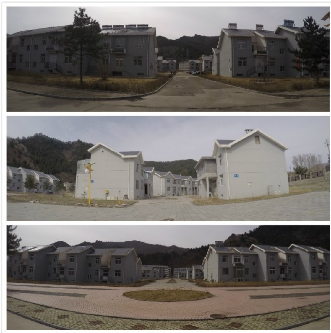
Figure 12: New dwellings for relocated families from Taihuai in Jingangku Township
