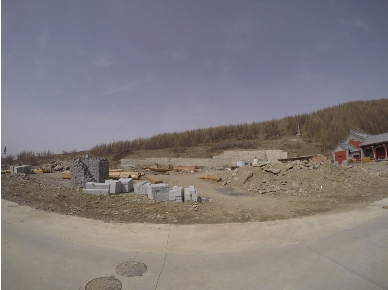
Figure 9: Yuhua Monastery is under reconstruction
