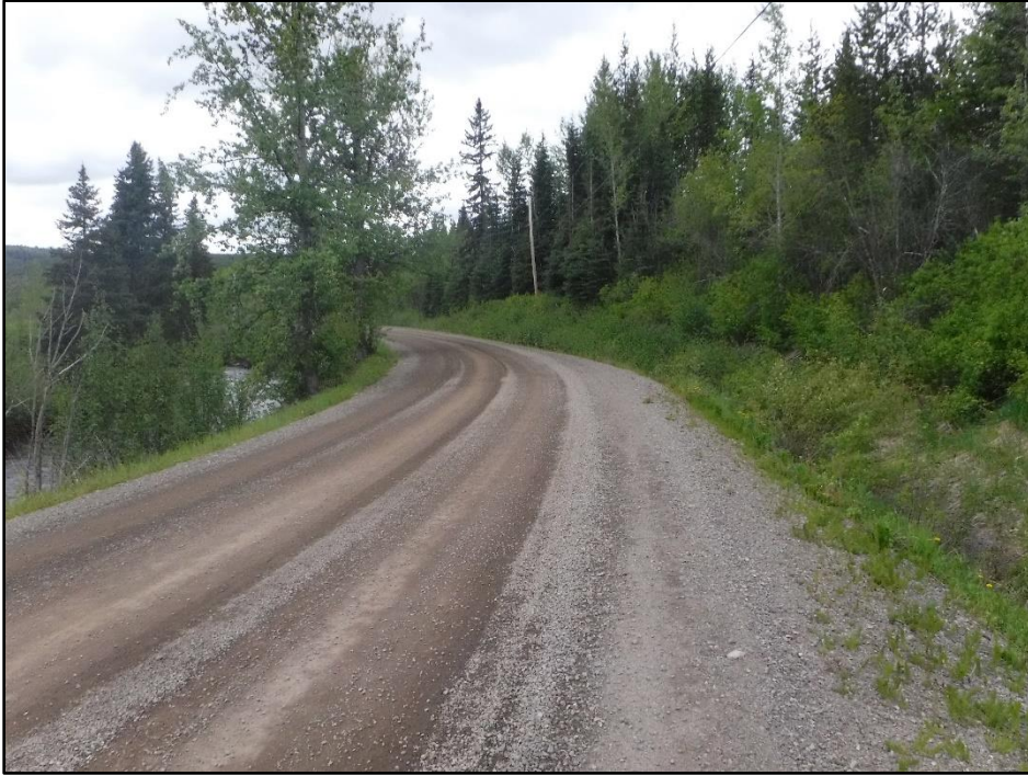
Figure 2.11. Redistribution of coarse materials across a road surface (sweeping).
