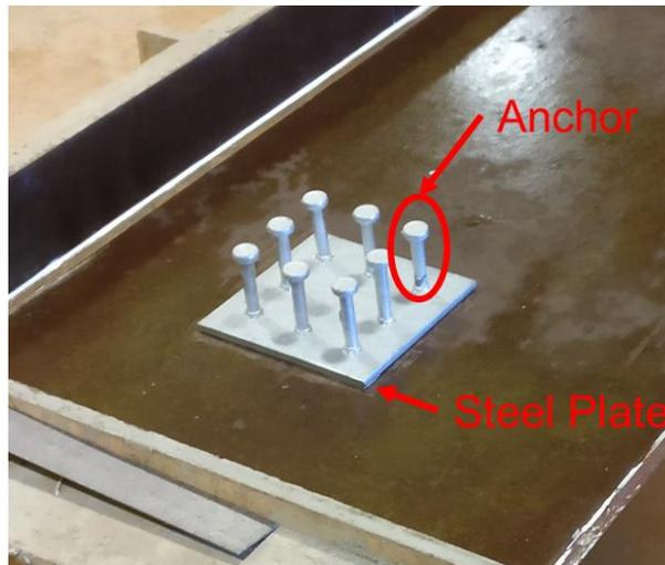
**Figure 1.3 Embedded plate with welded headed stud anchors**
