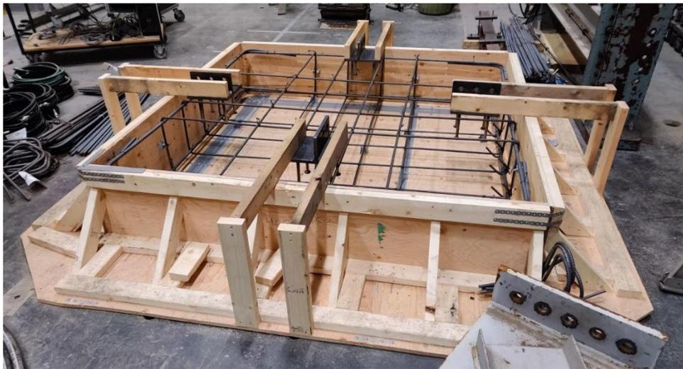
**Figure D.4 Installation of SEP4 embedded plates**
