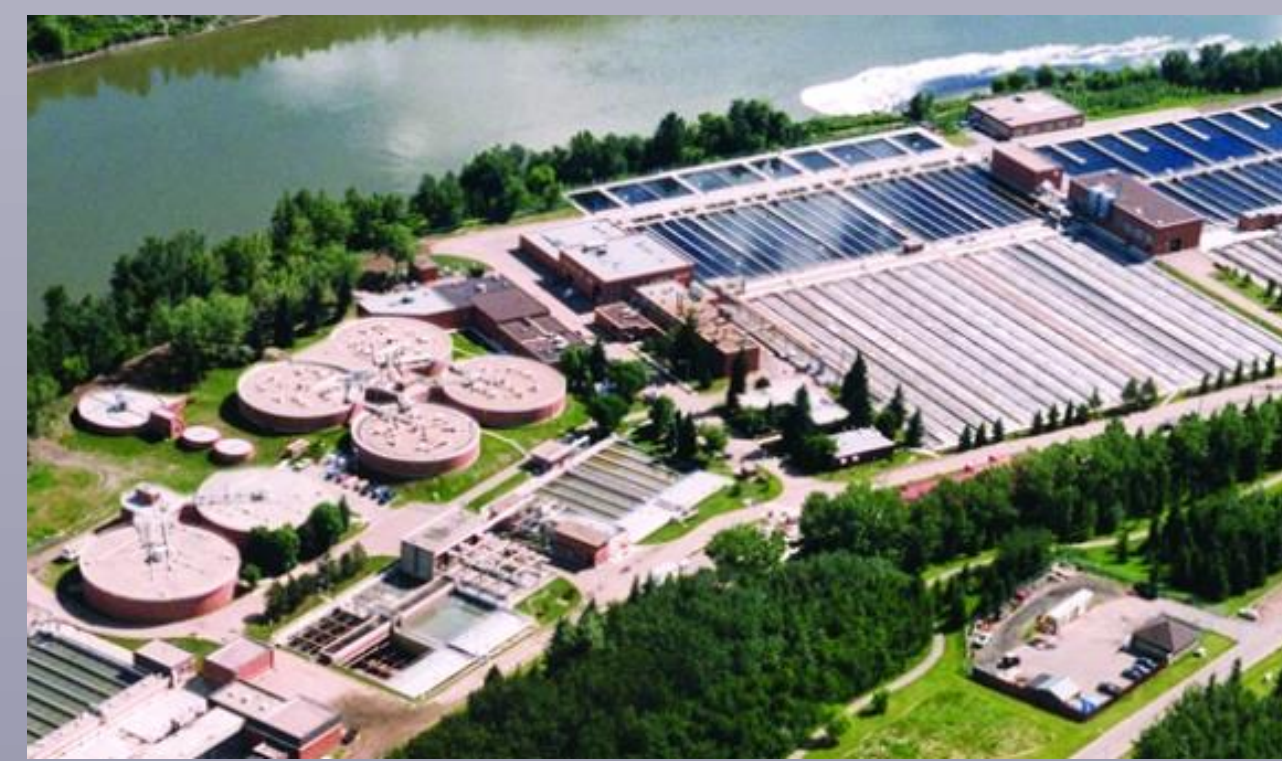
Figure 1.2 Aerial view of the Goldbar Water Treatment plant, Edmonton, Alberta 6
