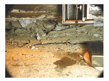
(b) a view of crack in footing cover concrete on north side of the column
