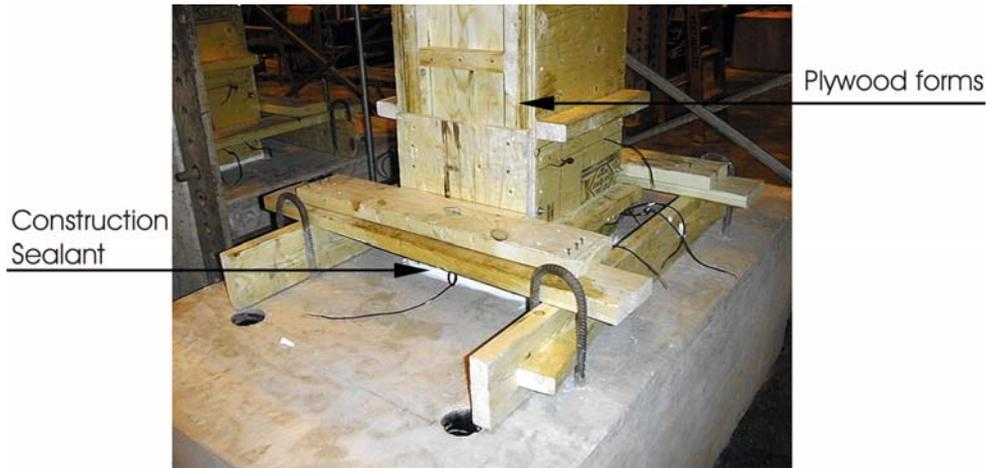
Figure 4-5: Construction sealant applied at potential location of leakages
