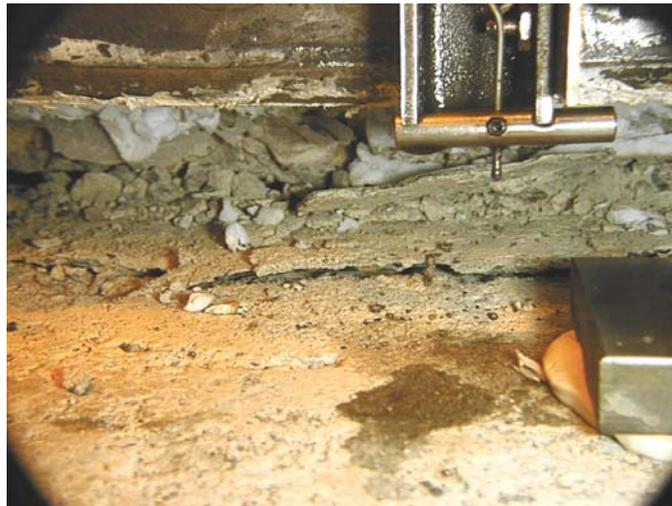
(b) a view of crack in footing cover concrete
