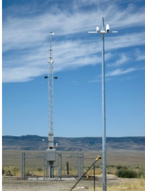
Figure 1. A typical RWIS station
