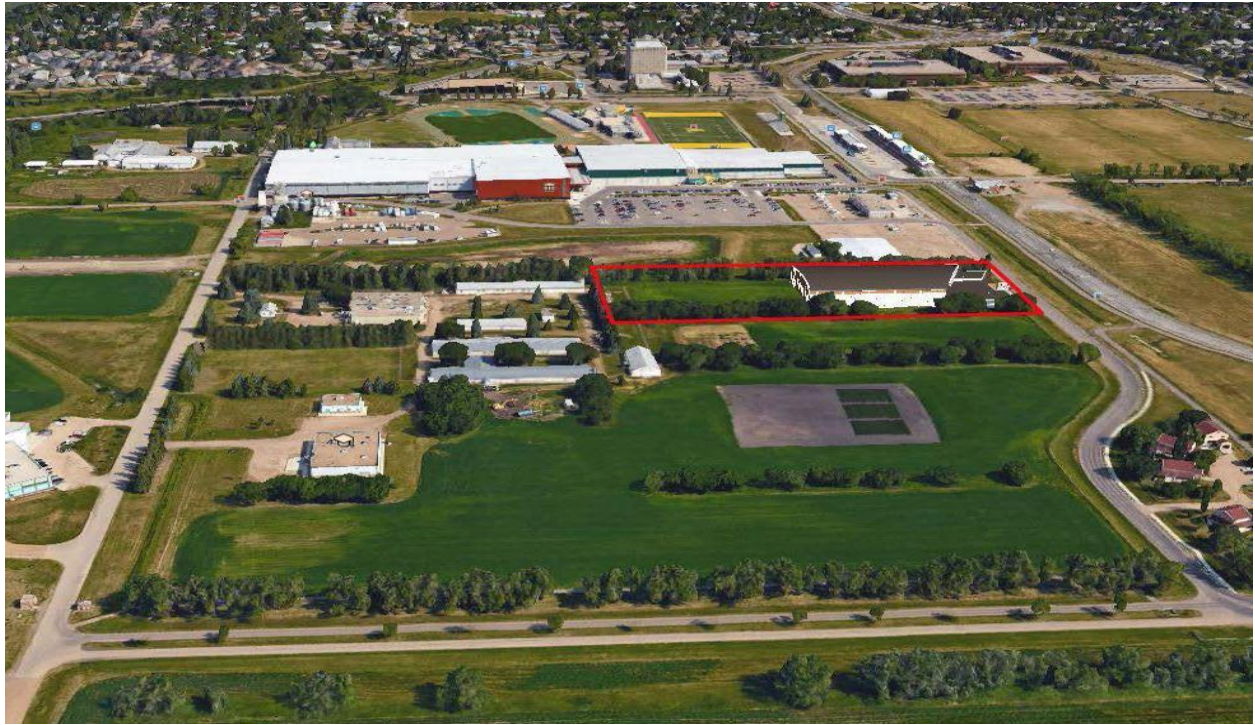
Fig. 1. Aerial photograph showing proposed RCRF building and site (outlined in red). University of Alberta. RCRF Design Development Report submission – January 11, 2016. Stuart Olson/HFKS Architects, Inc.
