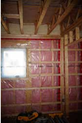
Figure 3.48: Exposed wall assembly with Insulation (FG-MDa Architects)
