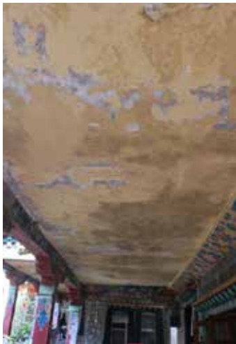
Figures 5.34 and 5.35: Roof leakage and water damage to the painted detailing of a column and capital (W Semple)
