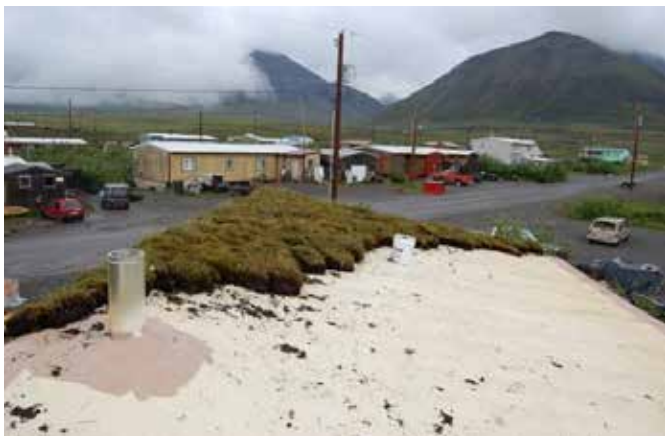
Figure 3-32 and 3-33: Berming the house, and Installing sod on the roof (CCHRC)
