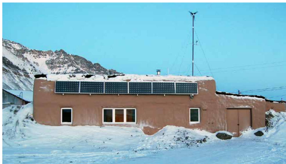
Figure 3-34: Completed Prototype Home with solar and wind installations (CCHRC)
