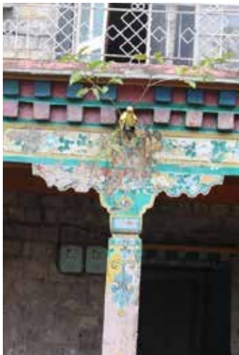
Figures 5.34 and 5.35: Roof leakage and water damage to the painted detailing of a column and capital (W Semple)
