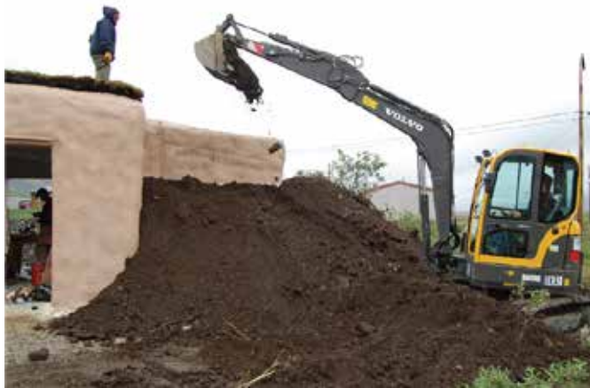
Figure 3-32 and 3-33: Berming the house, and Installing sod on the roof (CCHRC)
