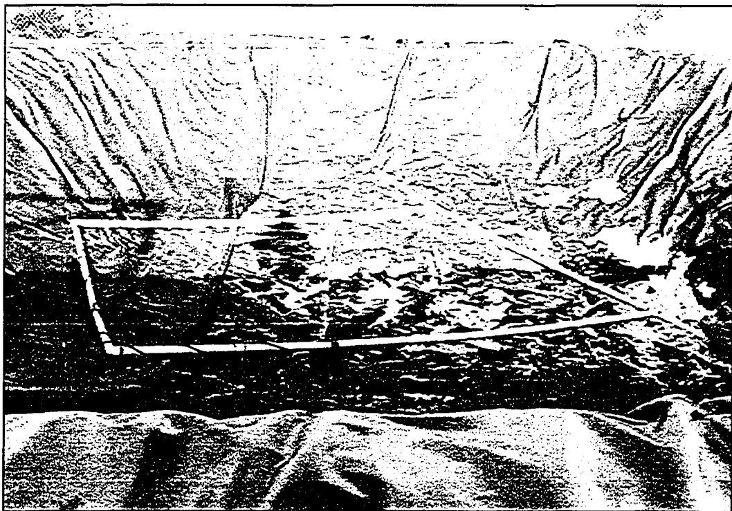
Figure 2.5 Collection system piping prior to placement of gravel and sand drainage layers.
