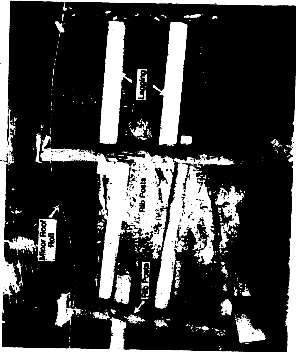
Plate 16. NEWLY EXPOSED PILLAR SIDE AND SUPPORTS
