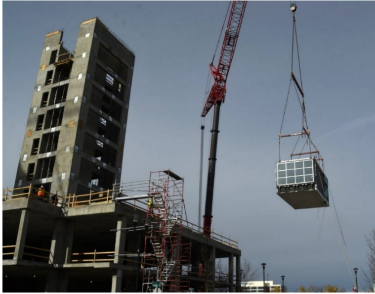
Figure 1.4: Modules assembly for ALT Hotel in Calgary, Alberta (Cappis 2017)
