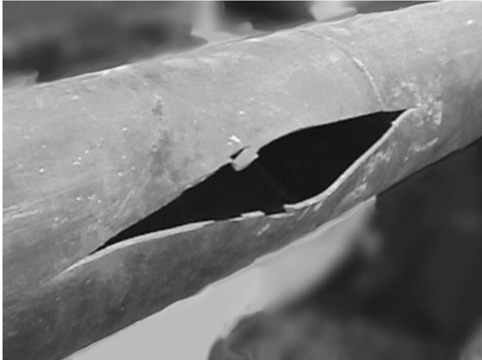
Figure 1.3 Failure of an oil pipeline 800 m downstream of a pump station [11]
