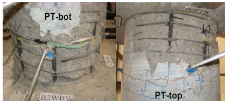
Figure 2.12. Damaged state partially post-tensioned bent (Cruz Noguez et al. 2012)
