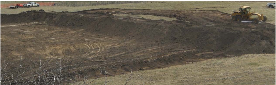
Figure 6-13 Grader for haul road maintenance
