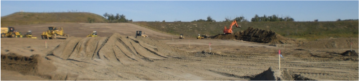
Figure 6-12 Fill and compact process
