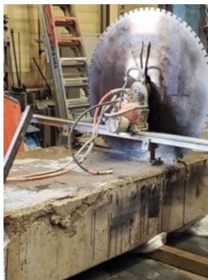
Figure 4- 8: Flexural girder cutting.
