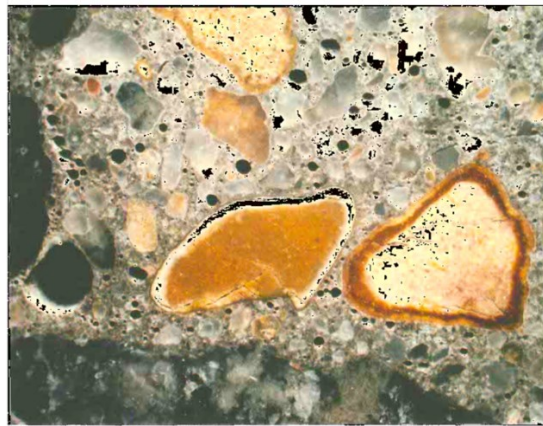
Figure 2- 2: ASR within the concrete (darkened rim on granite gneiss and chert particles by ASR) (Lane, 1994).
