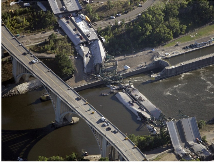
Figure 2- 4: Collapsed I-35W bridge in Minneapolis, MN (Gash, 2007).
