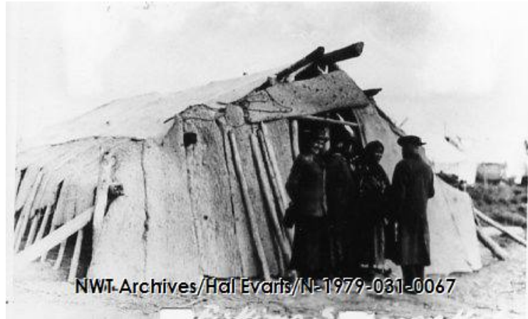
Figure 8. Anglican Bishop Isaac O. Stringer visits an Inuvialuit camp near Teet'it Zheh or Tsiigehtshik. This structure was made from aatr'ii. Dinjii Zhuh anthropologist explains that "large pieces of bark are peeled from trees in the spring when the sap is running and used as shingles and siding for smokehouses." 59 Aatr'ii provides good temperature regulation in the smokehouse. Untitled, undated, c. 1920s. Archival Caption: "Bishop Stringer of the Anglican Mission Yukon and Northwest Territories at Eskimo summer camp at either Fort McPherson or Arctic Red River. The sides of this camp are sheets of spruce bark peeled from spruce trees." 60
