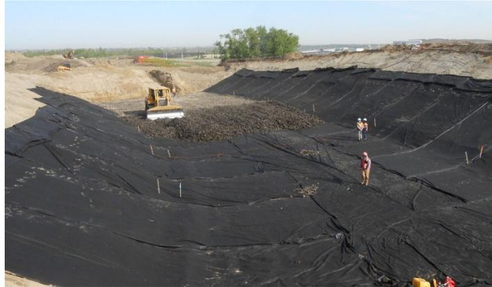
Figure 4.4: Excavation for test embankment covered with geotextile at the bottom and on the side slopes.
