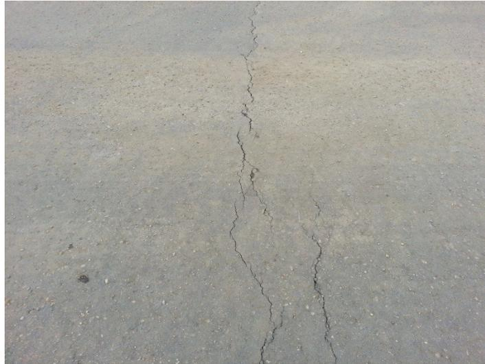
Figure 5.3: Photo of transvers crack observed at the start of the PLTT section.
