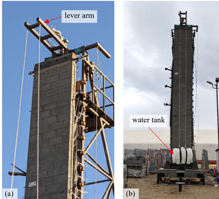
Figure 4.13: Vertical load application system (a) Chains connected to the lever arm on top of the structure (b) Suspended water tank used to apply vertical loads.
