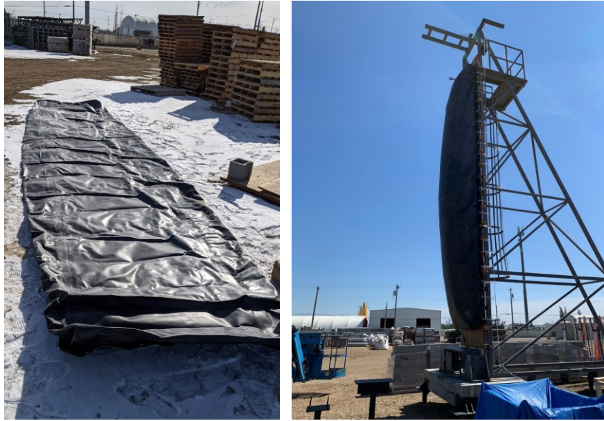
Figure 4.20: Airbag (a) Before installing (b) Installed and fully inflated.
