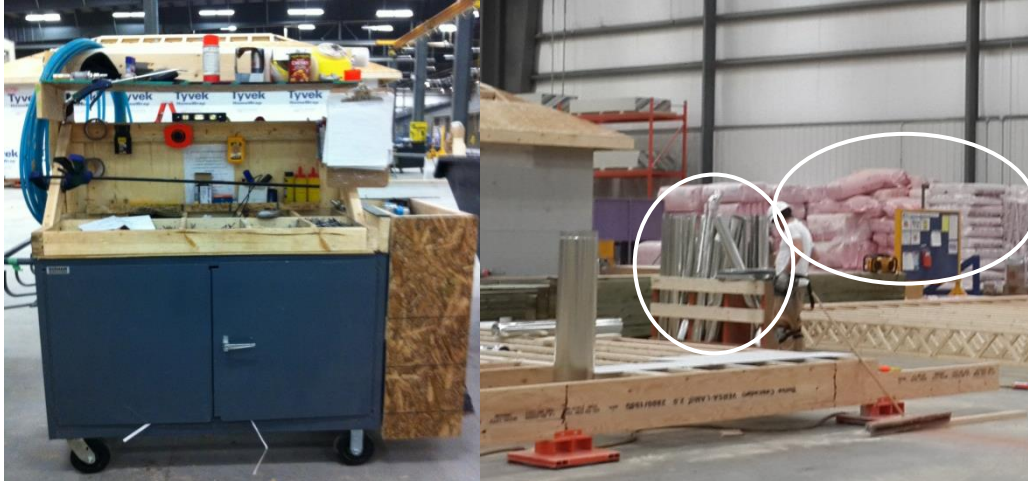
Figure 54: Portable work-carts and material staging point
