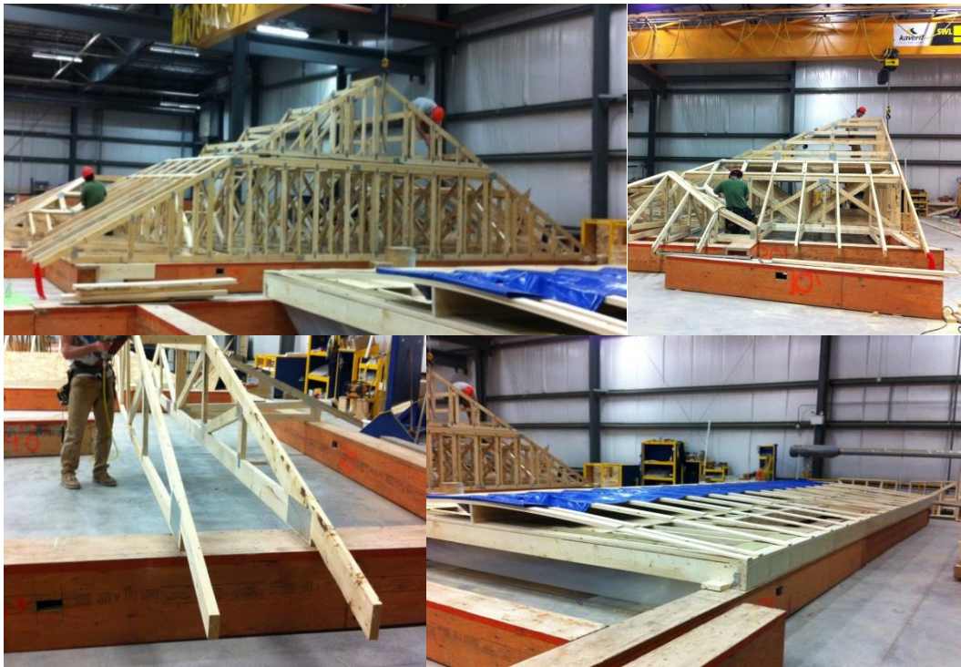
Figure 62: Roof station – existing platform to frame roof/ceiling
