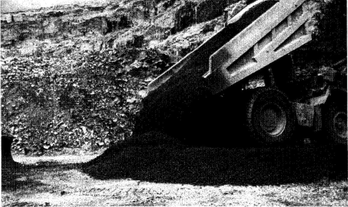
Figure 4.19 Dumping of subsequent load after compaction of previous CRF
