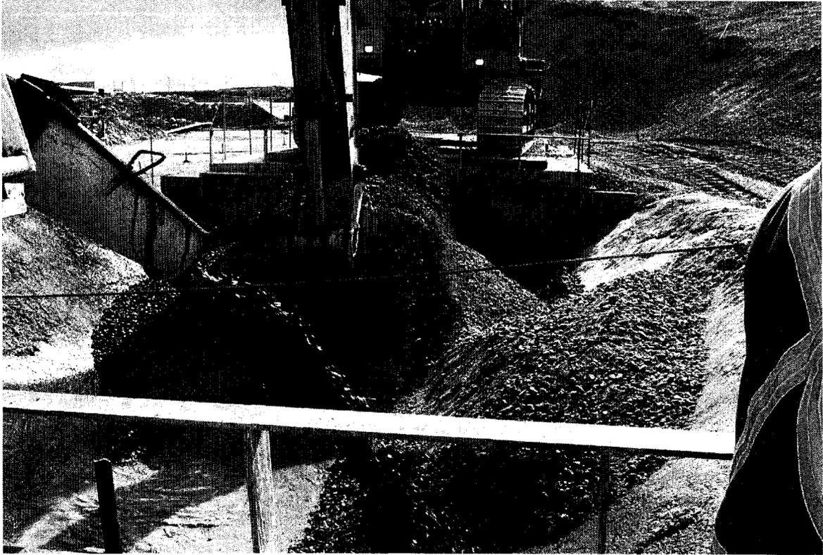
Figure 4.8 Pouring of cement slurry, and mixing it with aggregate by excavator
