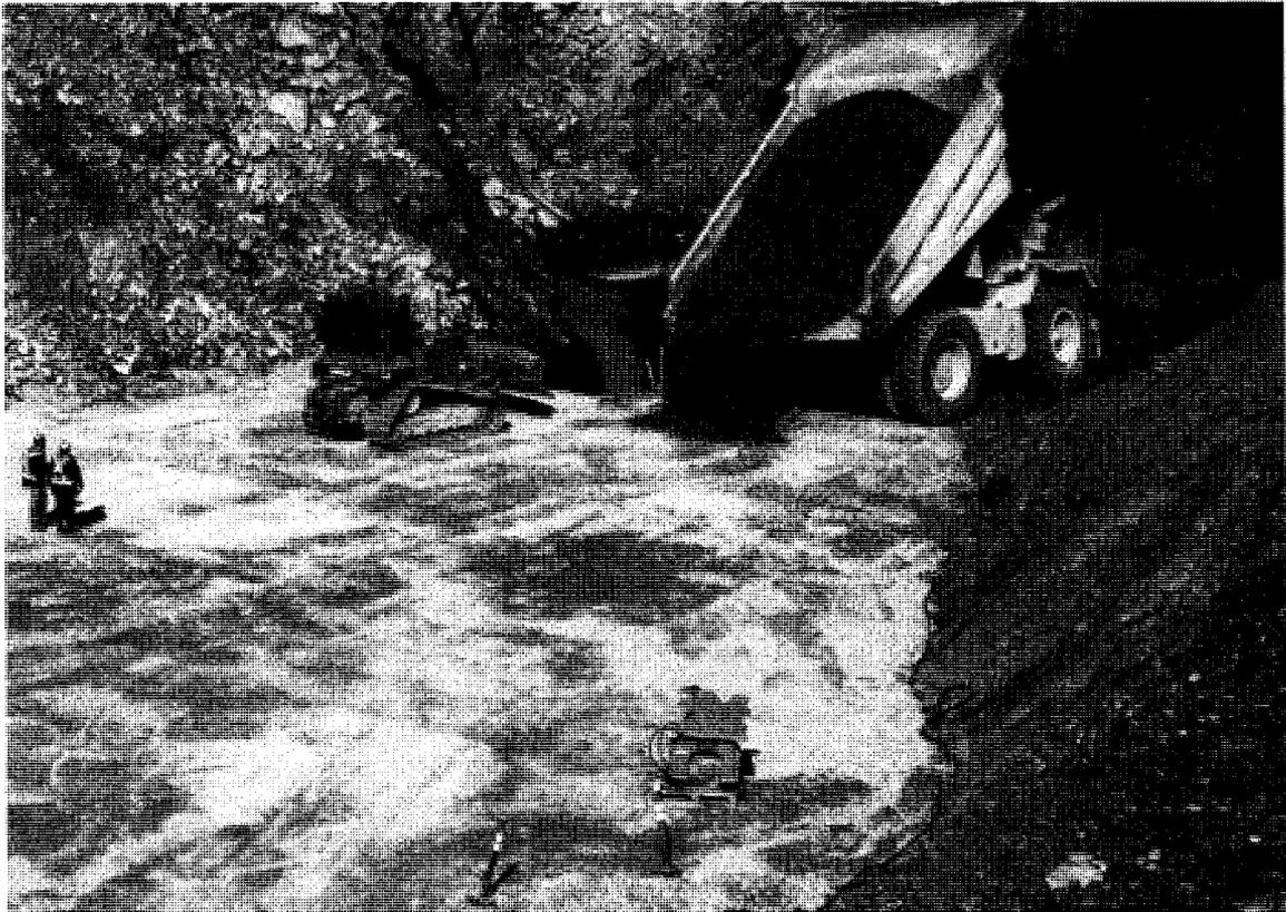
Figure 4.17 CRF is being dumped at placement area by Cat 777 haul truck
