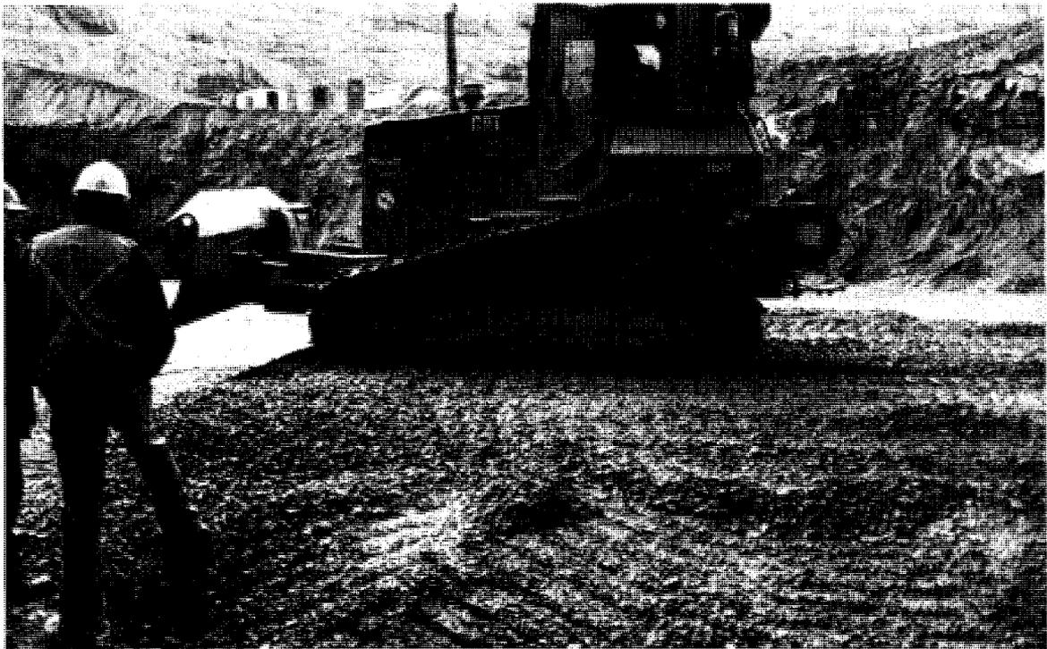
Figure 4.20 Spreading and compaction of CRF in first lift in progress
