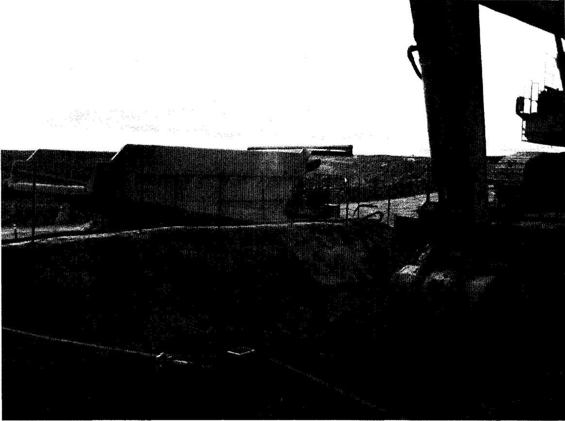
Figure 4.10 Mixed CRF ready to be loaded into haul truck
