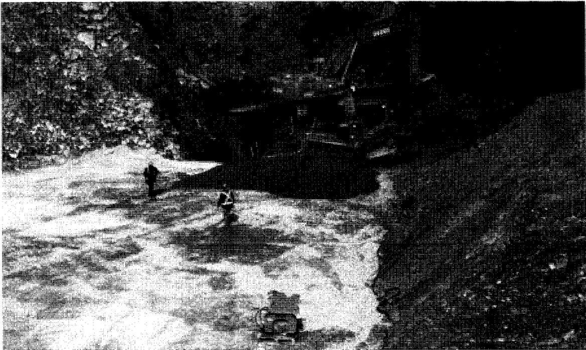
Figure 4.18 Spreading of CRF by a dozer
