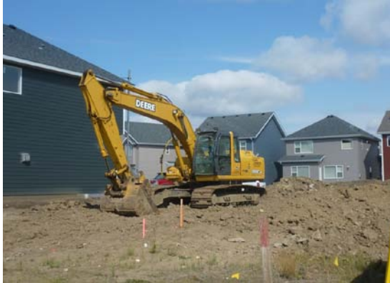
Excavation of site
