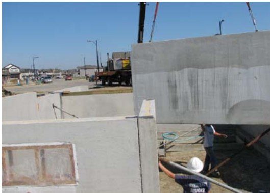
Crane lifting wall panel
