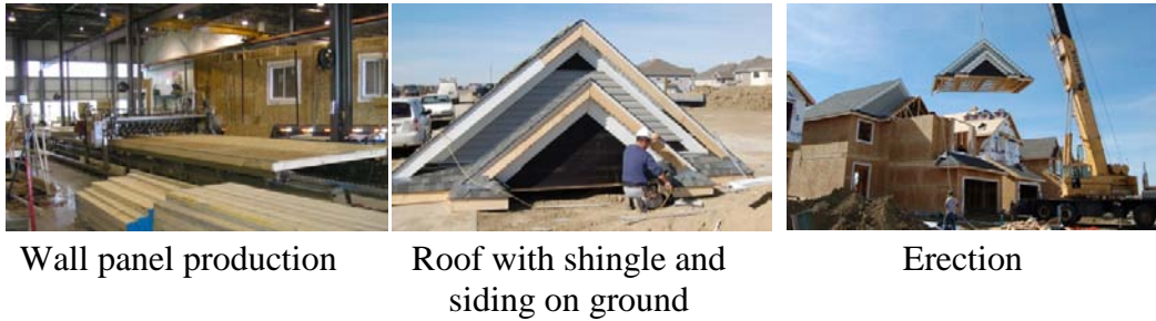
Figure 2.19: Photographs of Panelized Construction
