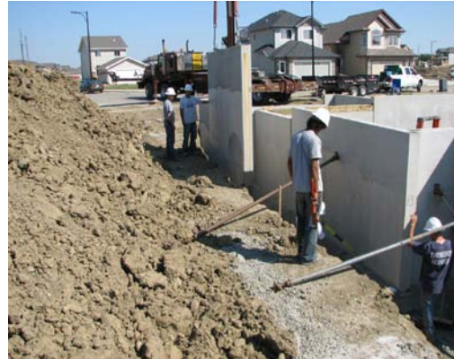
Wall section placement
