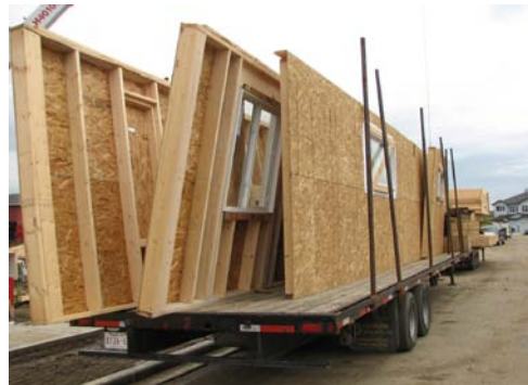
Shipping wall panels
