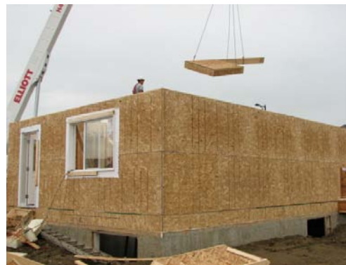
Assembly of wall panels
