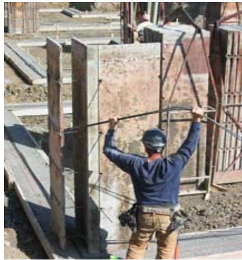
Foundation wall form preparation
