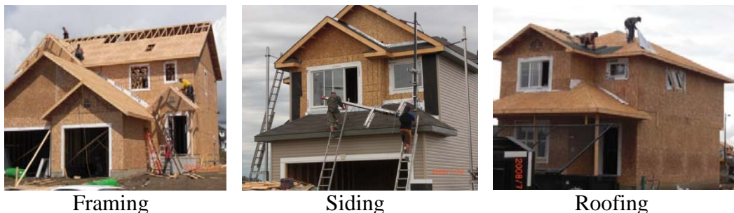
Figure 2.18: Photographs of Onsite Built Method
