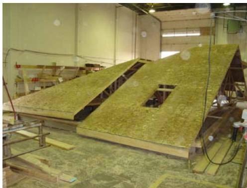
Roof section at fabrication shop
