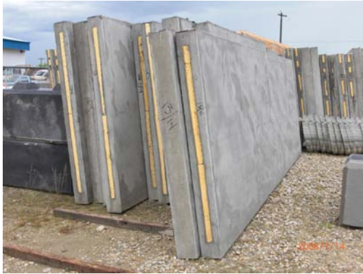
Pre-Cast wall panels delivered to site
