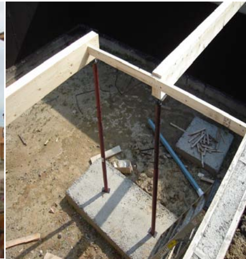
Foundation grade beam installation
