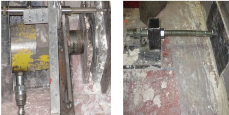
Figure 3.23 – Mechanical fixation at the bottom of Oan's walls (2013)
