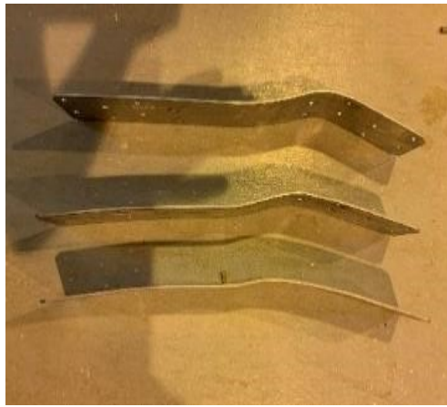
a) Deformation of steel plates of panel joint connections
