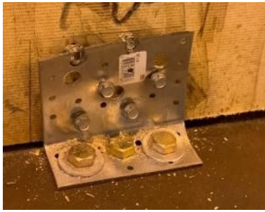
(c) Shear out failure.
