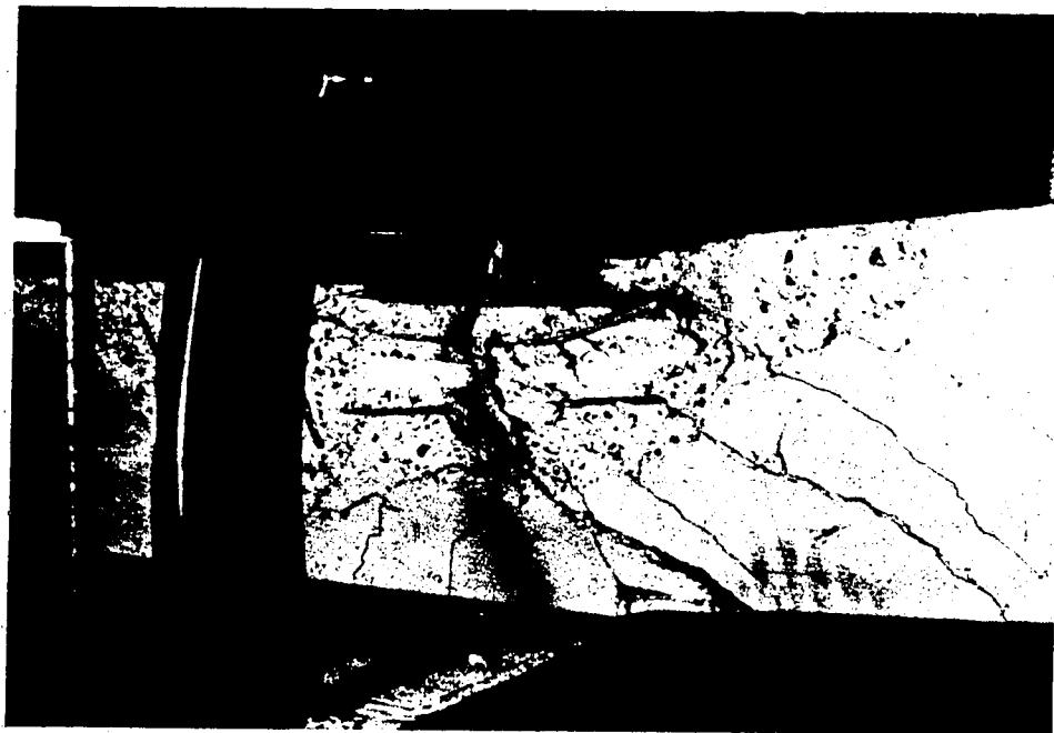
PLATE 5.2 LOCAL FAILURE OF BEAM T1
