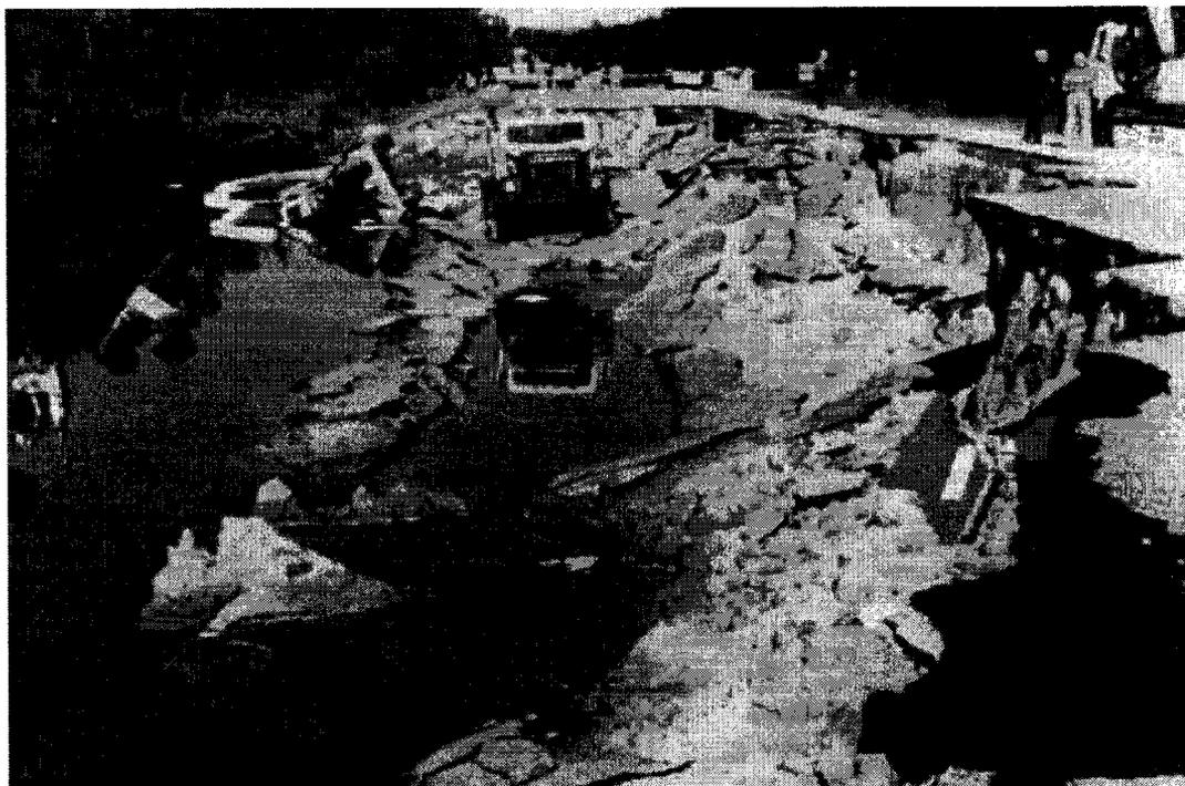
Figure B.32 Failure of the embankment on Ackerman Lake (After Hryciw et al. 1990)
